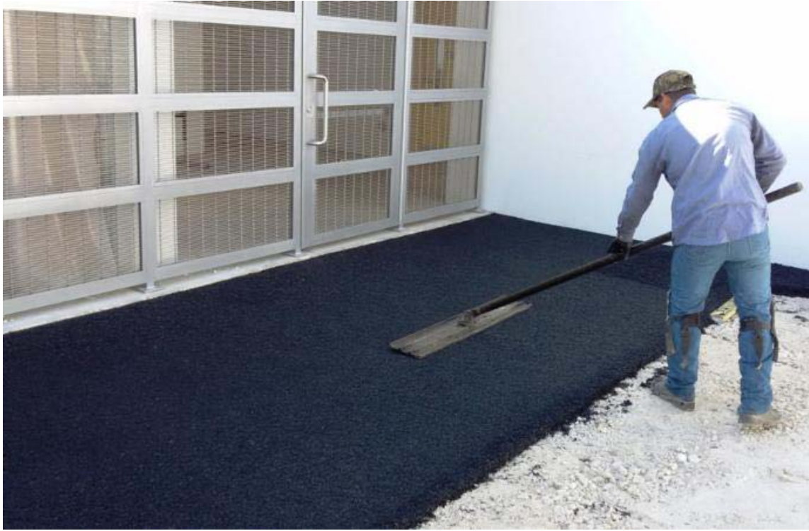
Top layer going on.
